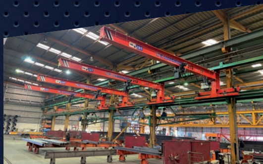
16 units, 1.6 t x 8 m, with Verlinde lifting equipment. Client: Liaromatis Facilities 2023, Patras Industrial Area
