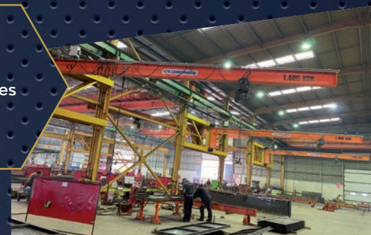
3,5 / 3,2 t x 9 m with Stahl lifting equipment. Client: Liaromatis Facilities 2004, Patras Industrial Area
