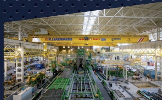
32/5 t x 41.4 m, with Demag lifting equipment. Client: Teka Systems 2021, Oinofyta, Boeotia
