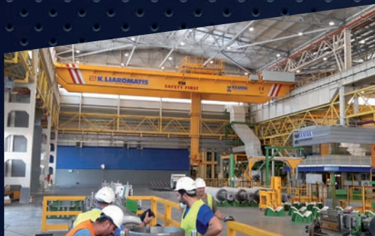
32/15 t x 41.4 m, with Verlinde lifting equipment. Client: Elval 2022, Oinofyta, Boeotia
