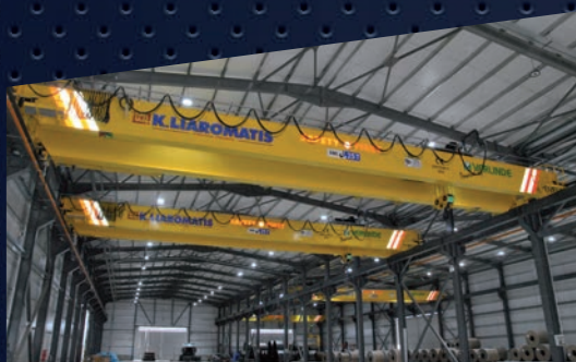
4 units, 25 t x 20.62 m, with Verlinde lifting equipment. Client: Vriko 2022, Aspropyrgos, West Attica
