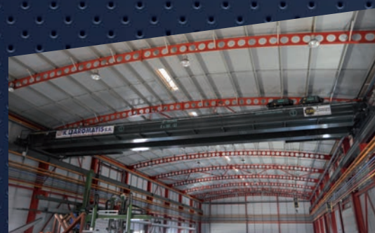
2 x 20 t x 26 m, with Verlinde lifting equipment Client: Liaromatis Facilities 2007, Patras Industrial Area
