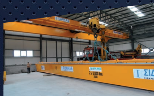
2 x 8 t x 29 m, with Verlinde lifting equipment. Client: Sidma Steel 2011, Oinofyta, Boeotia
