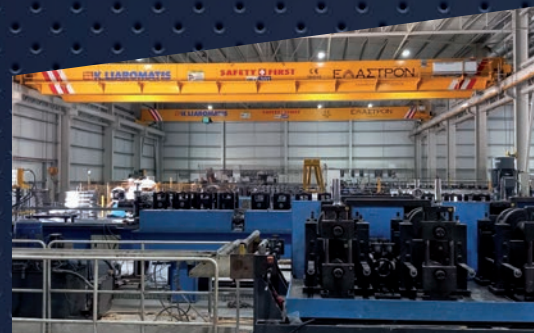
20 t x 24.35 m, with Verlinde lifting equipment. Client: Elastron 2022, Aspropyrgos, West Attica
