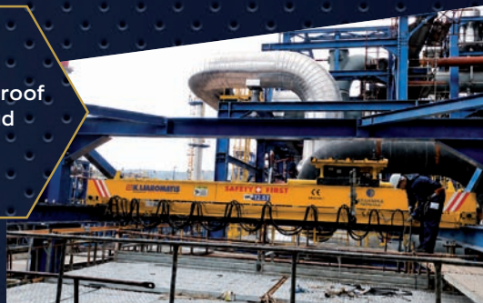
Top-running double-girder crane, 5 t x 12 m, with Verlinde lifting equipment. Client: Hellenic Petroleum 2015, Aspropyrgos, West Attica
